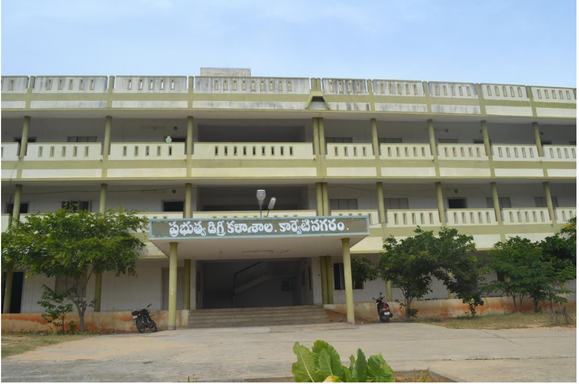
Front View of College Building Government Degree College, Karvetinagaram.
